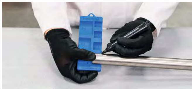
Figure 28 – Marking the insertion depth
