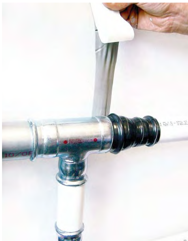
Figure 38 – Protection of the connectors with butanol adhesive tape
