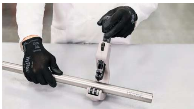
Figure 25 - Cutting the pipe to length
