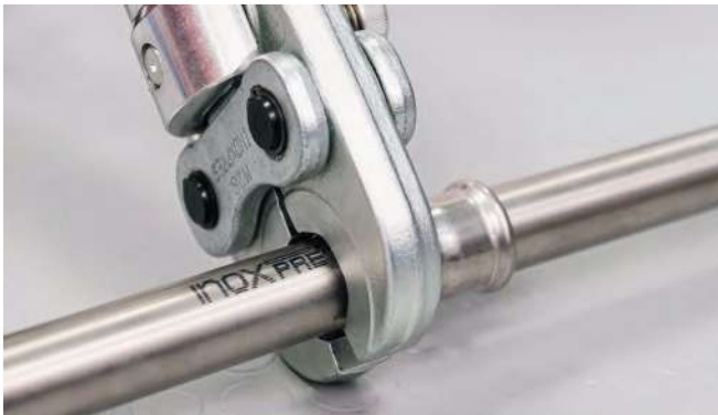
Figure 32 - Making the press connection
