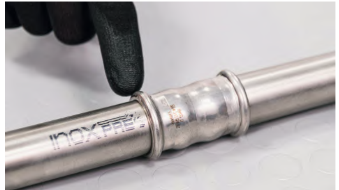
Figure 33 - Checking the press connection
