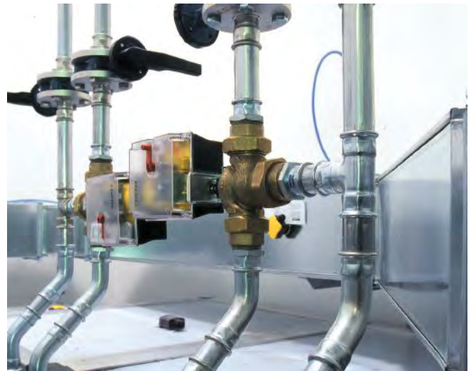
Figure 22 - steelPRES - refrigeration (closed circuit)
